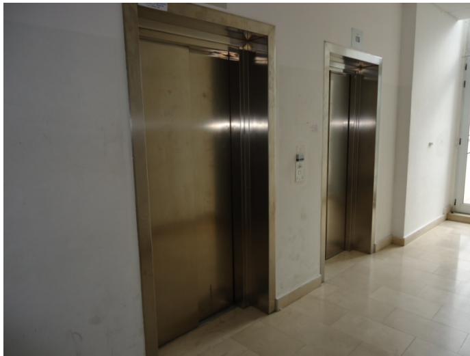
Picture 6 : FESB Elevators
