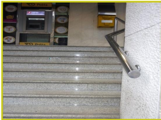
Picture 34 : Handrail and stairs
